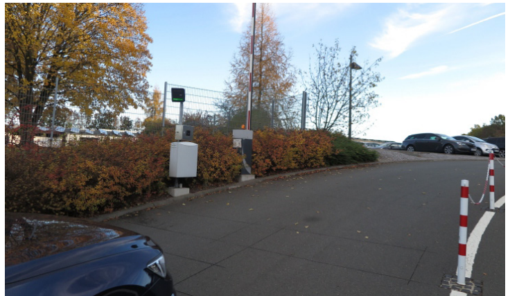
Parking Management: Comfortable access without waiting
